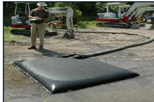
Plate 3-2 Silt Bag under inspection
